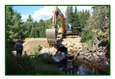
Finally, with regard to maximum physical slope at a crossing, Enviro Span can be installed as steeply as the side slope of the subgrade. Essentially, if the subgrade will remain stable at the point of crossing, then the Enviro Span installation will also remain stable.
